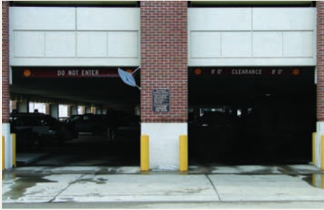
Photo 1: Example of Poor Informational Signage
